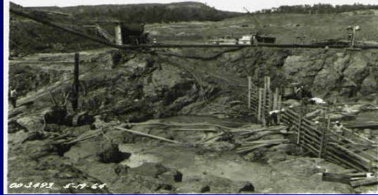
(Courtesy of California Department of Water Resources)
