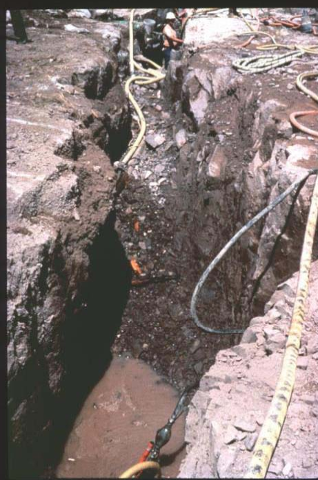
Upper Stillwater Dam Shear zone being cleaned out for concrete backfill
